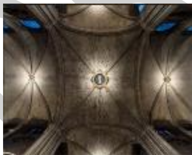
Figure (7): Ribbed vault [42]
