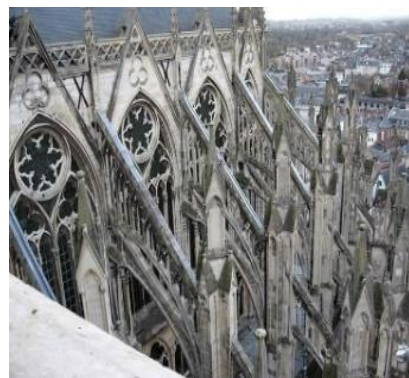
Figure (5): Flying buttresses [39].
