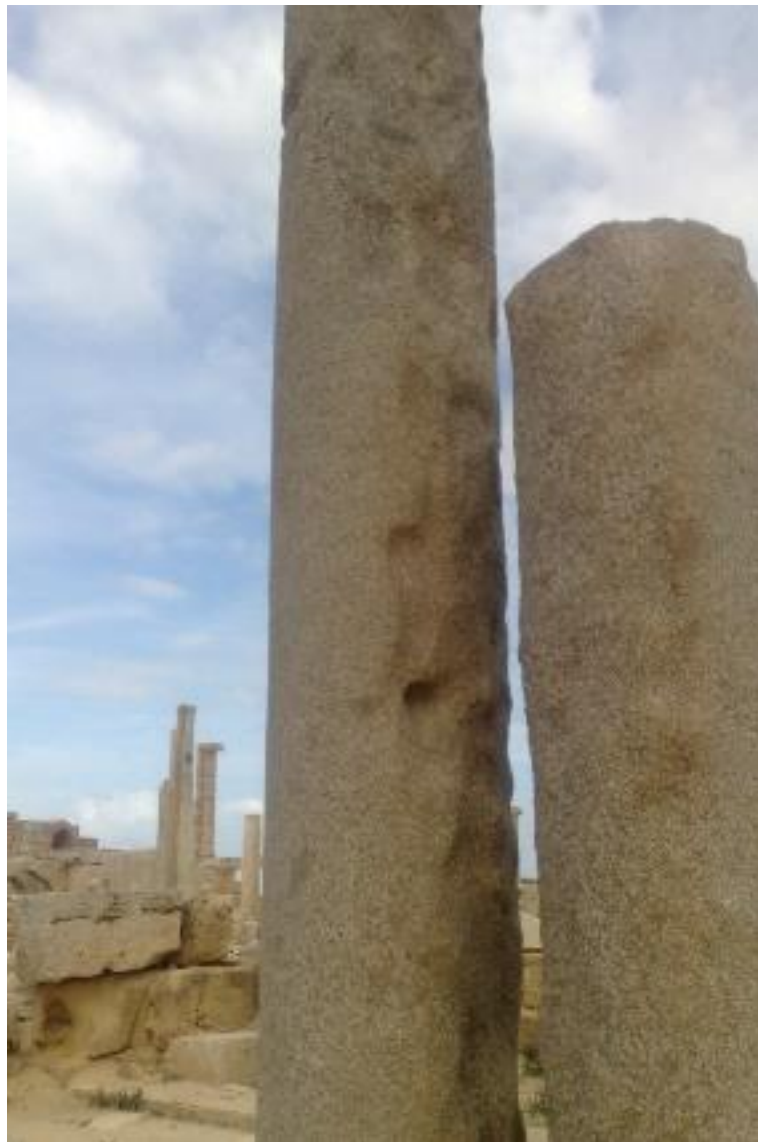
Figure (9): picture of the granite columns exposed to damage due to chemical weathering, direction of damage to the right of this image where the power station is located.
